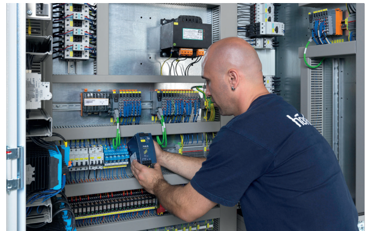
Control panel construction
